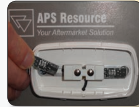
Inside LED Upgrade
