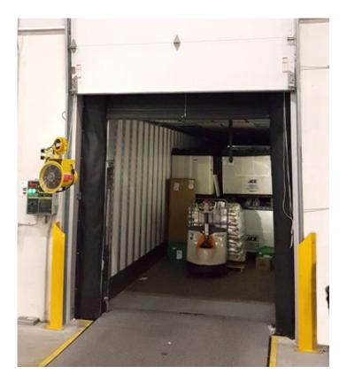
dock personnel comfortable working inside trailers as well as a High Impact LED™ Dock Light for increased visibility and energy efficiency. "We've found that the LED dock lights are a really stout design that can easily handle impacts from our 3-wheel forklifts," said Fischer.
