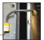
Interior dock lights can be powered through control panel and can be programmed to operate before dock operations begin.
